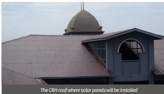
LTRU roof where solar panels will be installed
